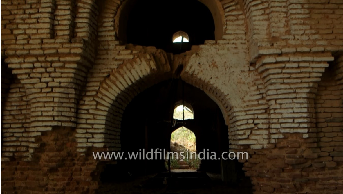
Broken arch inside Fort of Sheikhpur, Image Source: Image Source: (Youtube Channel: WildFilmsIndia)
